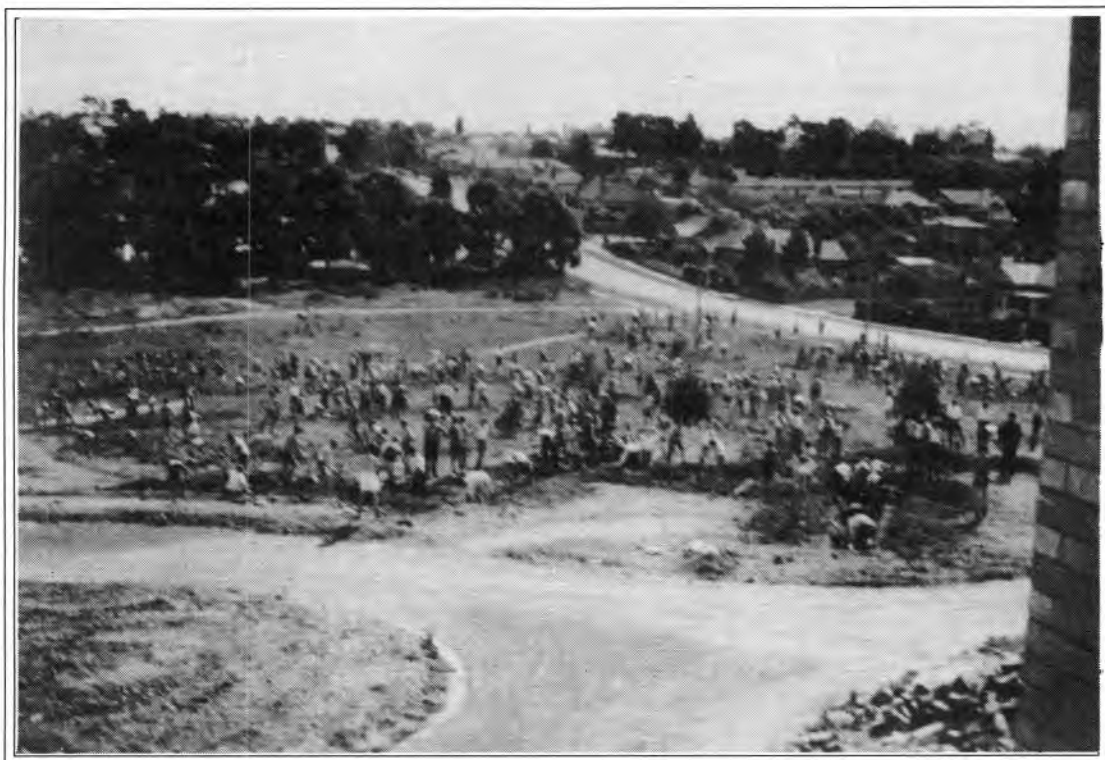
Digging air-raid trenches, early 1942 — boys at work. View taken from the front steps looking toward Prospect Hill Road.
